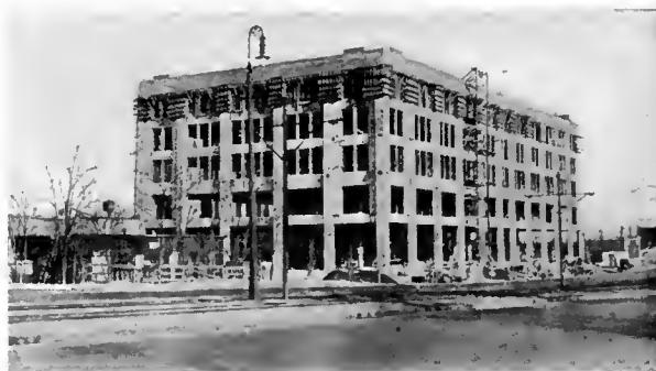
STRUCTURAL FRAME COMPLETED
